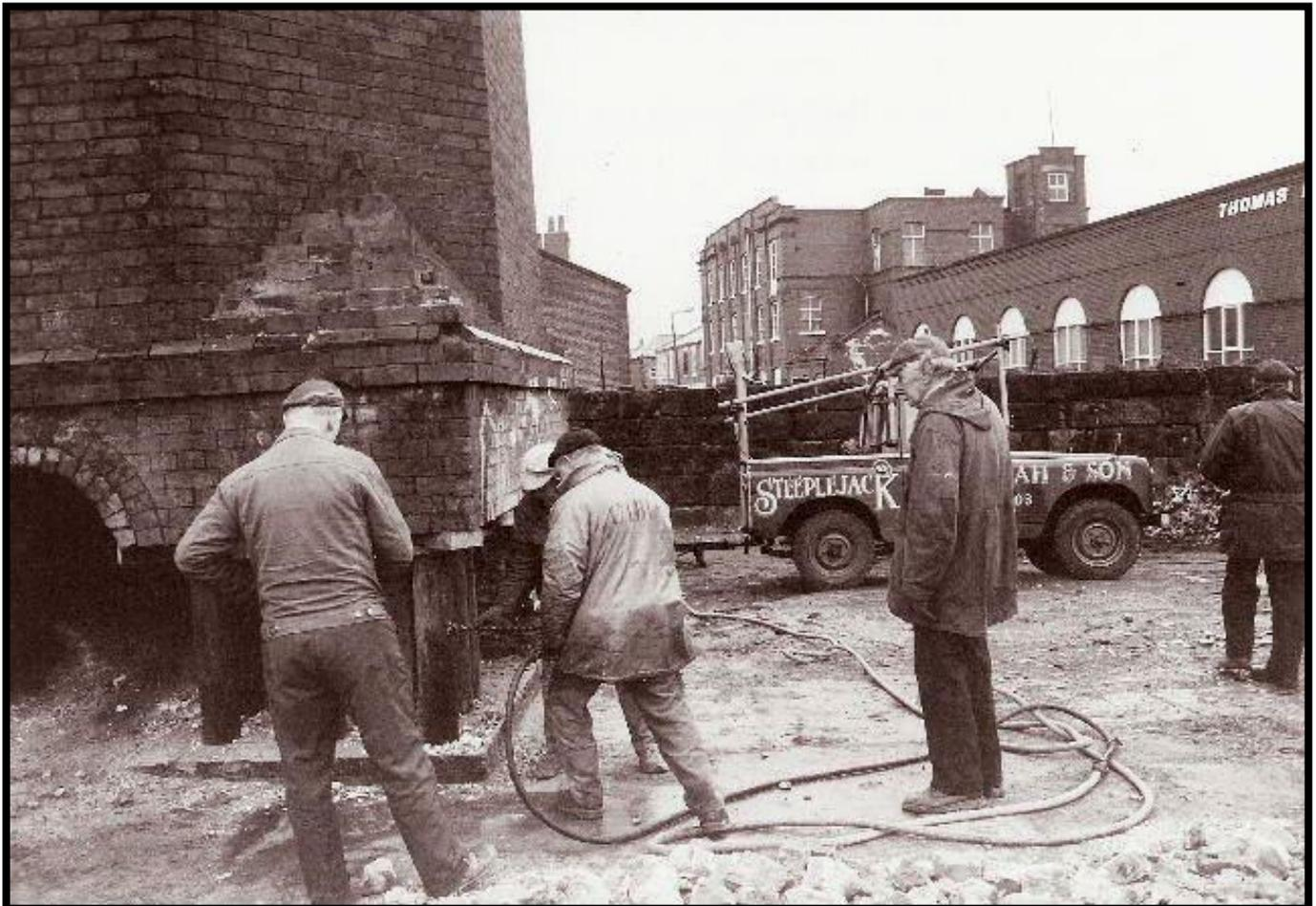
On the morning of the drop, Fred and fellow steeplejack Eddie Chattwood are hard at work boring holes into the pit props. These holes assist the flames to rapidly consume the timber. Notice to the left hand side the original flue. Fred's old Landrover workhorse, his 'Lanny' is parked to the rear.
